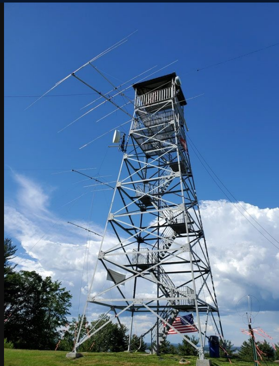
Stratham Hill Park fire tower — current Field Day site, with K1R antennas installed.
